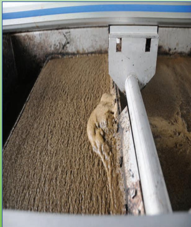
The combination of Ozone treatment process as a POME polishing plant, has been tested in operation for more than 9 months using the pilot R&D polishing plant, and results have shown to be able to treat the POME from the algae or aerobic pond discharge water to achieve the 20ppm BOD<sub>3</sub> limit.
